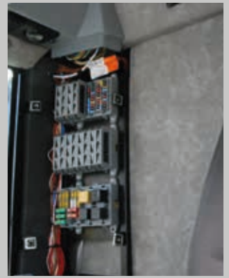
The electric fuses panel.
